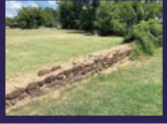
The ruins of the south side of the Historic Square in downtown Pilot Point.
